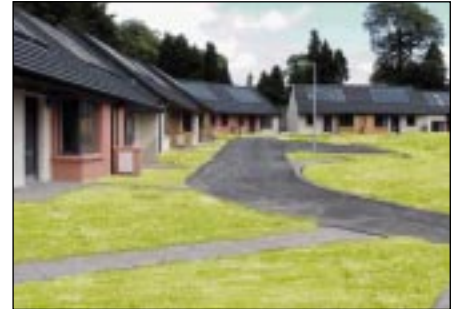
Some of the 26 high-tech / energy efficient Bungalows in St. John's Close.
